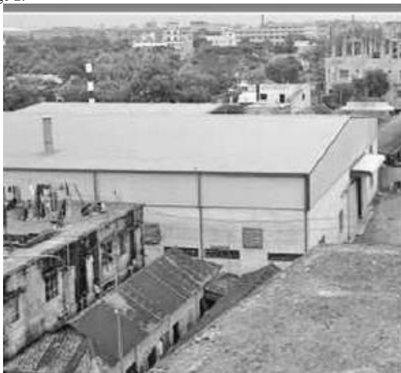
Figure 2: The proximity of the residential building and the factory
